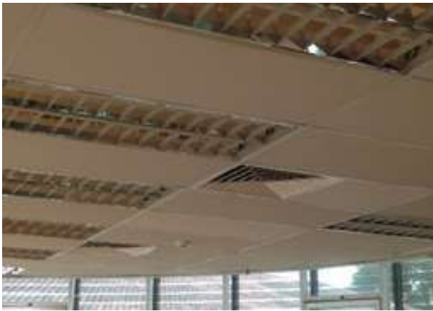
LED Lamp replacing conventional lamps
