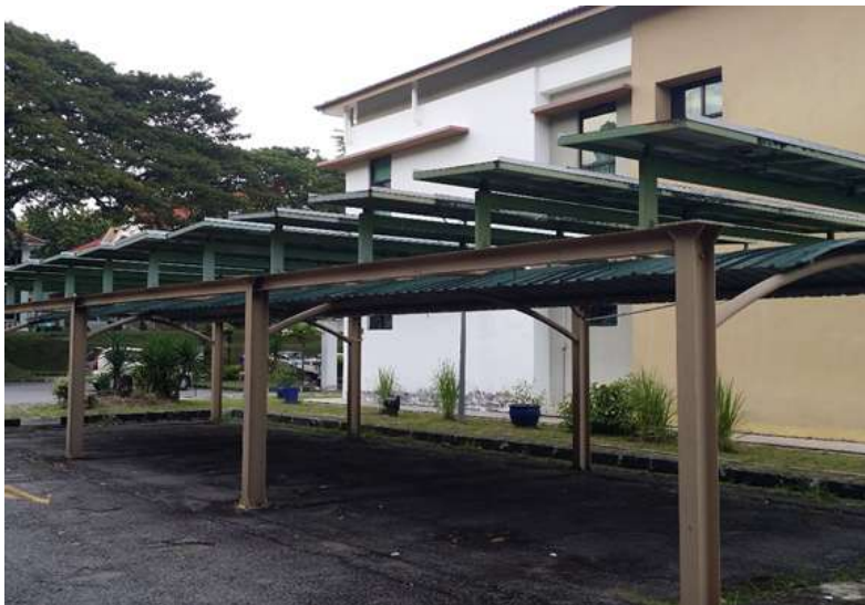
Solar Parking Lot (2.0 Kwh)
