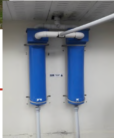
Rain Harvesting System at School of Humanities, USM
